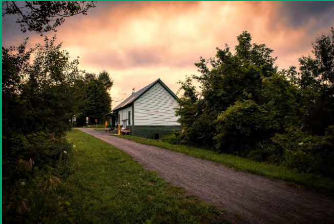
Danville Train Station
